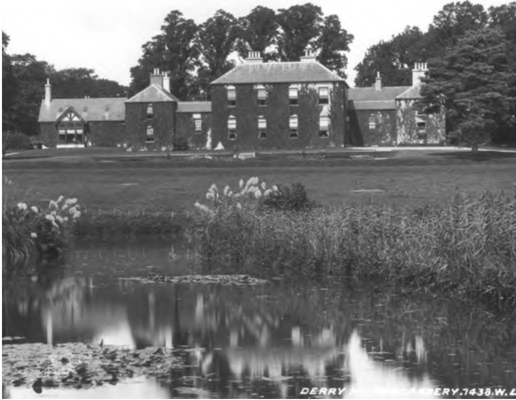
Derry ca 1900 Courtesy of the National Library of Ireland
